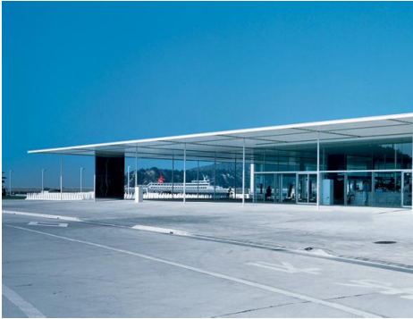
SANAA: Miyanoura port terminal
